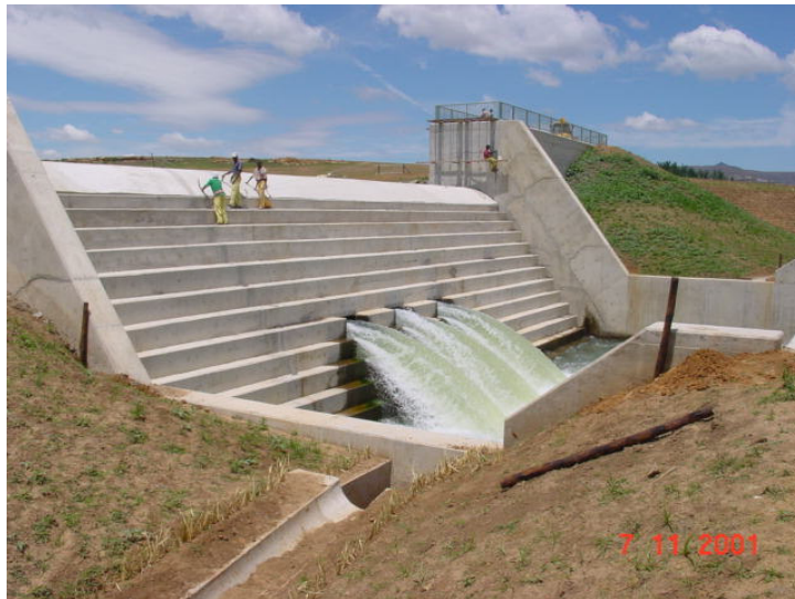
Figure 6. View of the Botterkloof Dam
